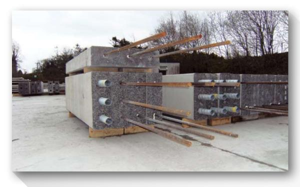
Precast Concrete Columns are generally considered for use on in-situ concrete flat slab projects where there's a high demand on tower crane hook time and tight construction programmes.
